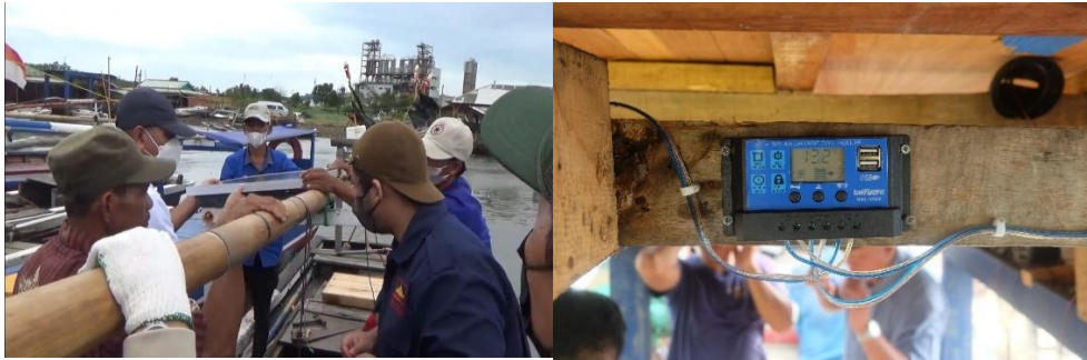
Figure 3. Training to Install Solar Panel Components
